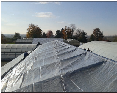
Changing the greenhouse roof
